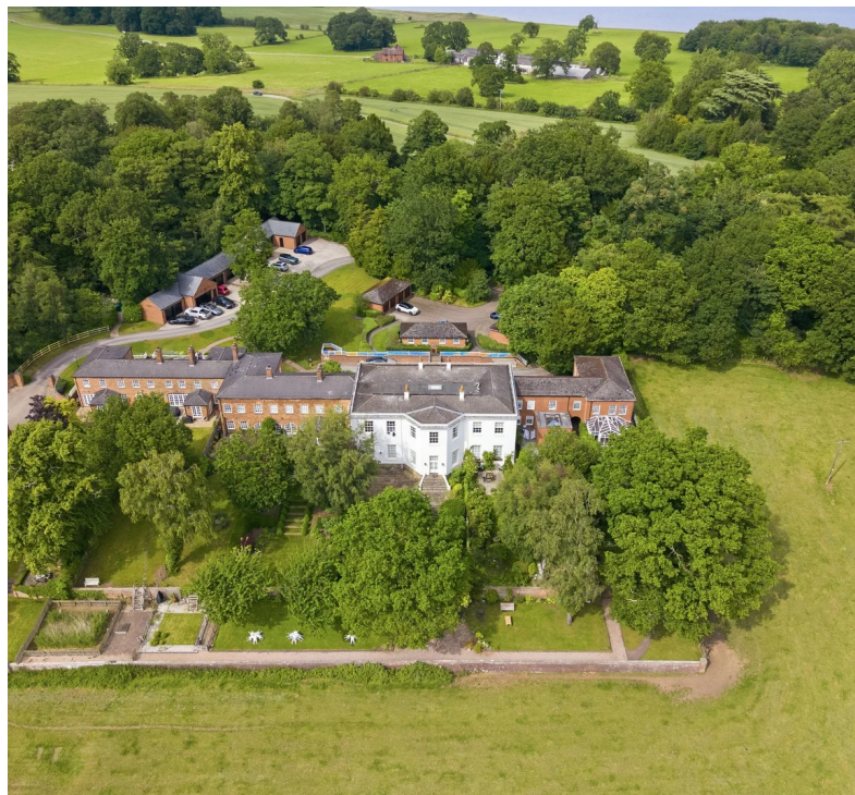
Ratford, The Old Rectory, Blithfield Hall Estate
